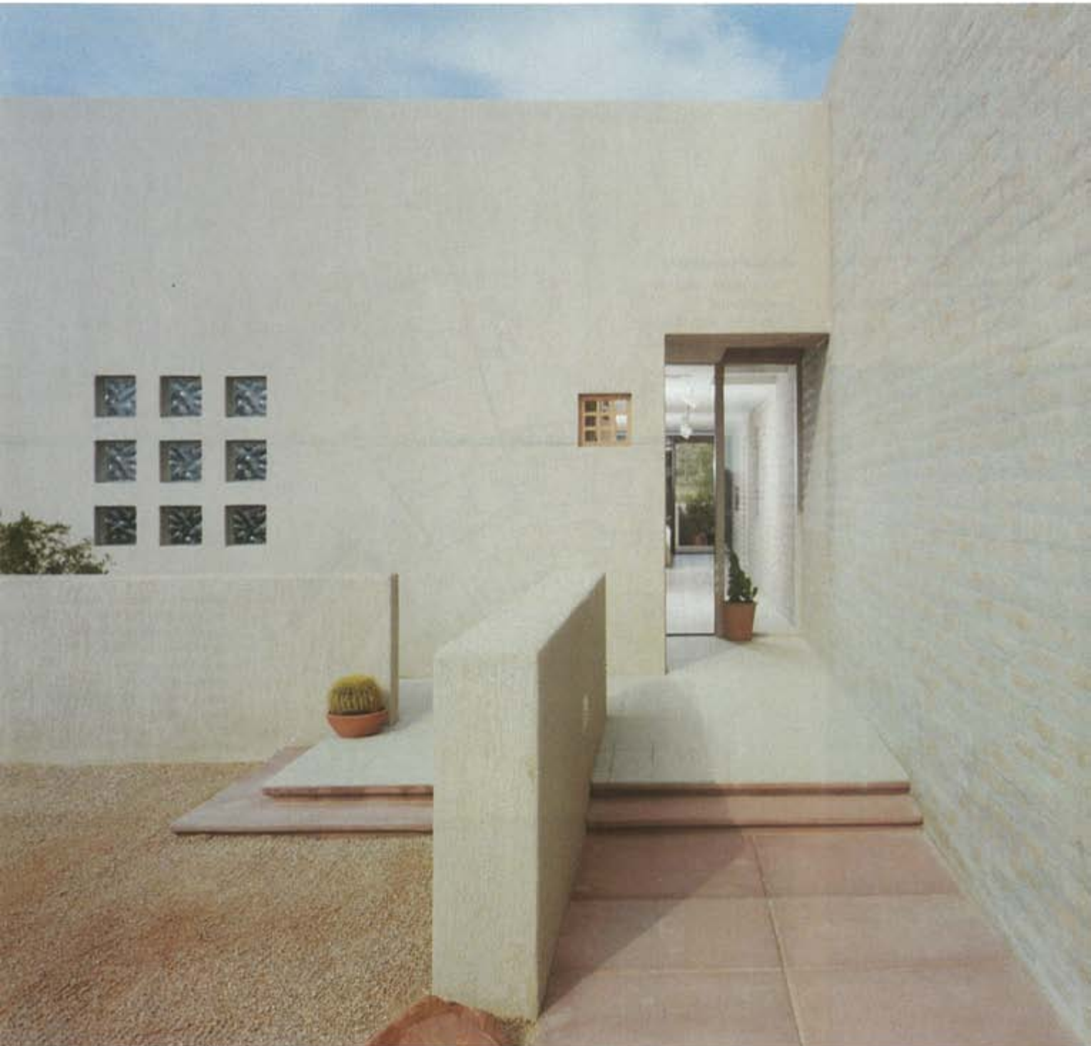
Above: The firm of Christensen Cassidy Billington & Candelaria created a contemporary expression of a Pueblo theme for the home of Rosalie and Louis Rosati in Mesa. The adobe-colored block wall defines the entry sequence and serves to organize the interior. Opposite page: The kitchen is the heart of the home and has easy access to a small office and studio loft. Photography by Neil Koppes.
